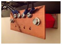
Figure 5. Ground bar Source: www.copper.org
